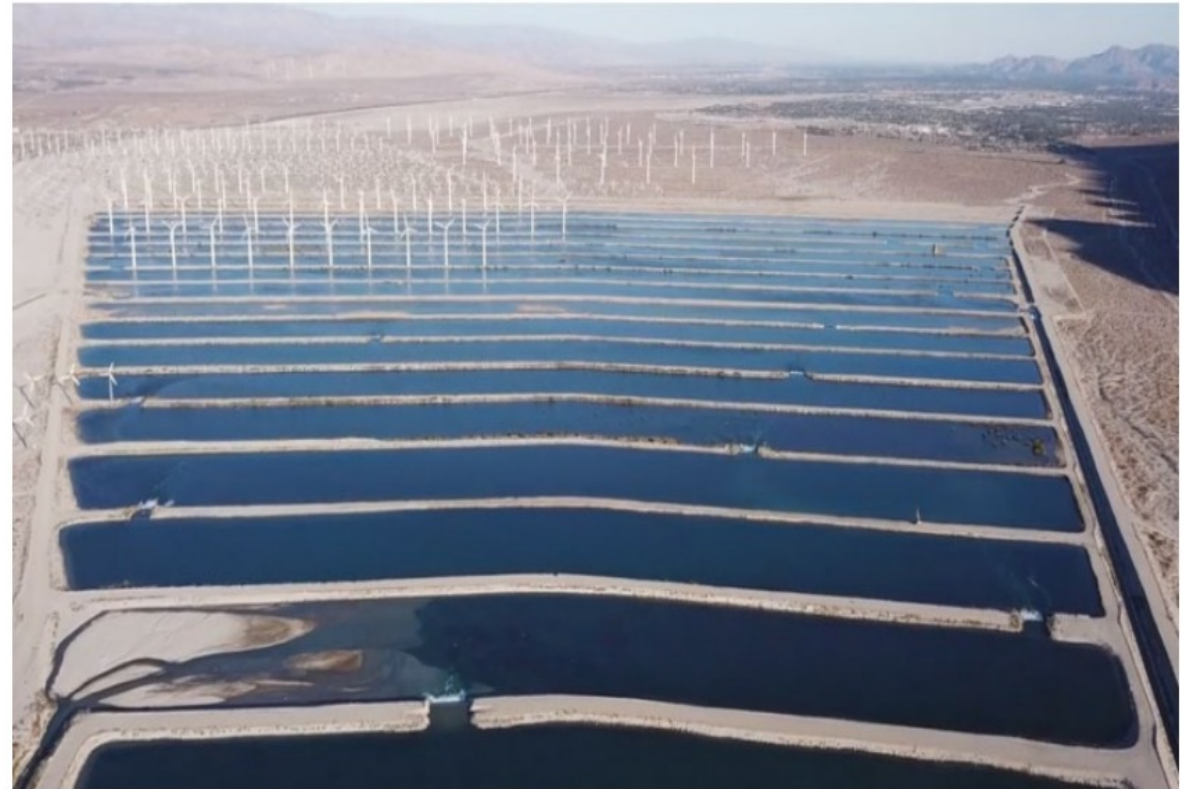
Imported surface water is recharged at the Whitewater River Groundwater Replenishment Facility
